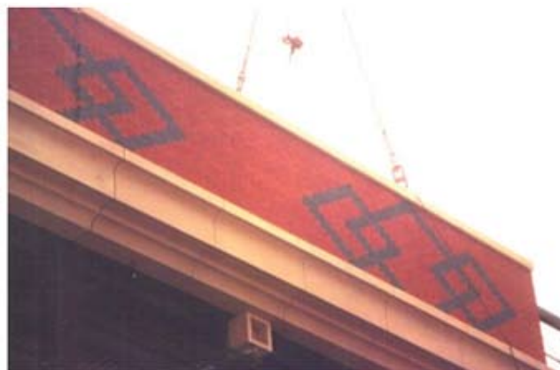
Project in Swansea using a cast-on finish of natural slate, and project in Manchester using brick (Photo: Trent Concrete Ltd)
