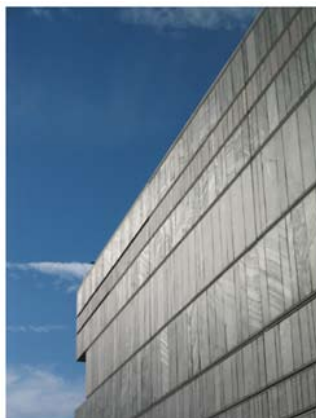
Project in Swansea using a cast-on finish of natural slate, and project in Manchester using brick (Photo: Trent Concrete Ltd)
