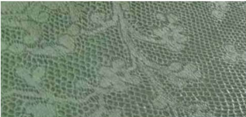
Project in Nottingham using a form liner to replicate lace. The image covers an area of concrete approx 300mm x 150mm. (Photo: Trent Concrete Ltd)
